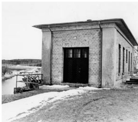
Pumpehus i Kolind Sund.
