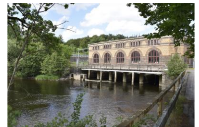
A small hydropower station in the south of Sweden.
