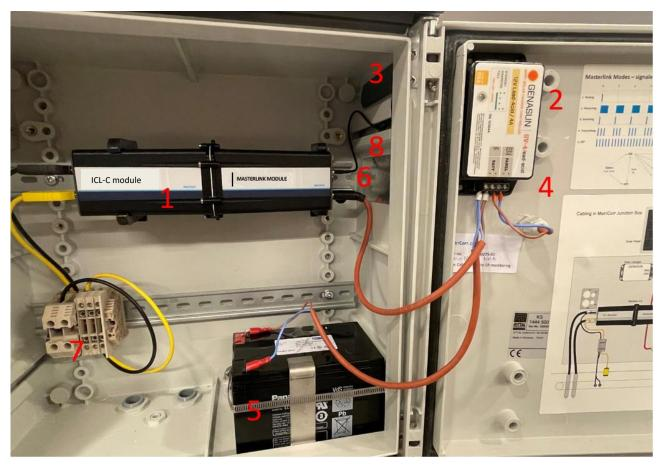
Figure 7: Interior of Solar Junction Box as Battery and solar connected.
