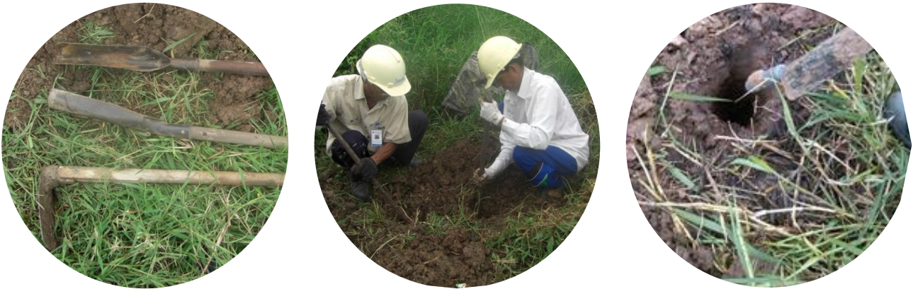
Hand digging using a dedicated set of specialized shovels and tools.
