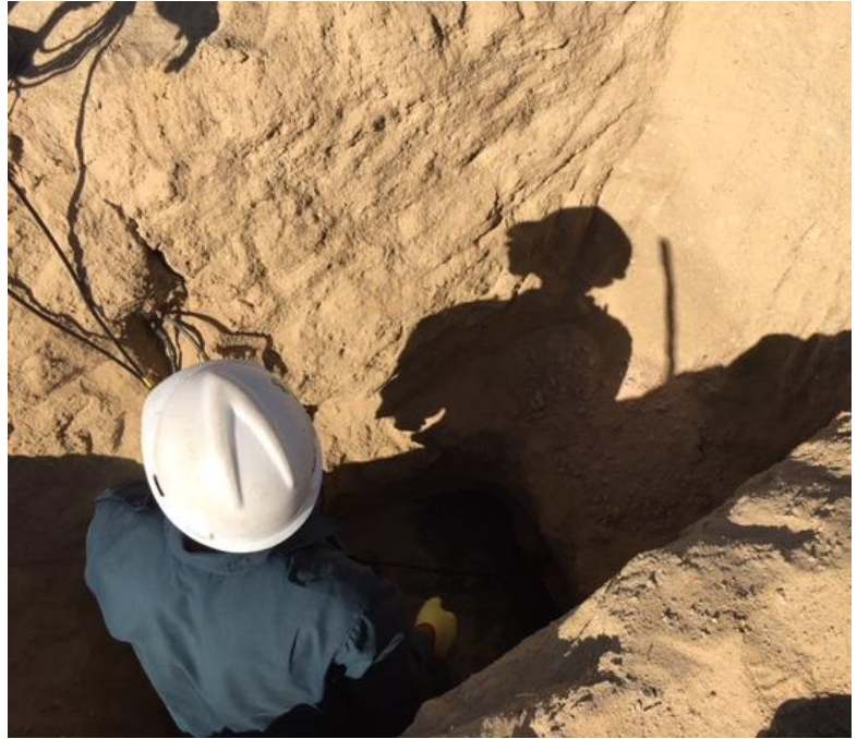
Hand-dig in the desert – full pipe excavation.
