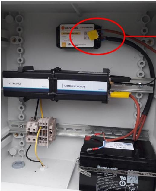
Step 3: Connect the Solar Charger OUT to the ICL power socket
