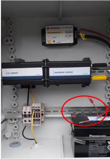
Step 1: Connect the Solar Charger to the battery
