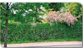
Acoustic fence made of steel, stone wool (core and acoustic material) and green PE netting
