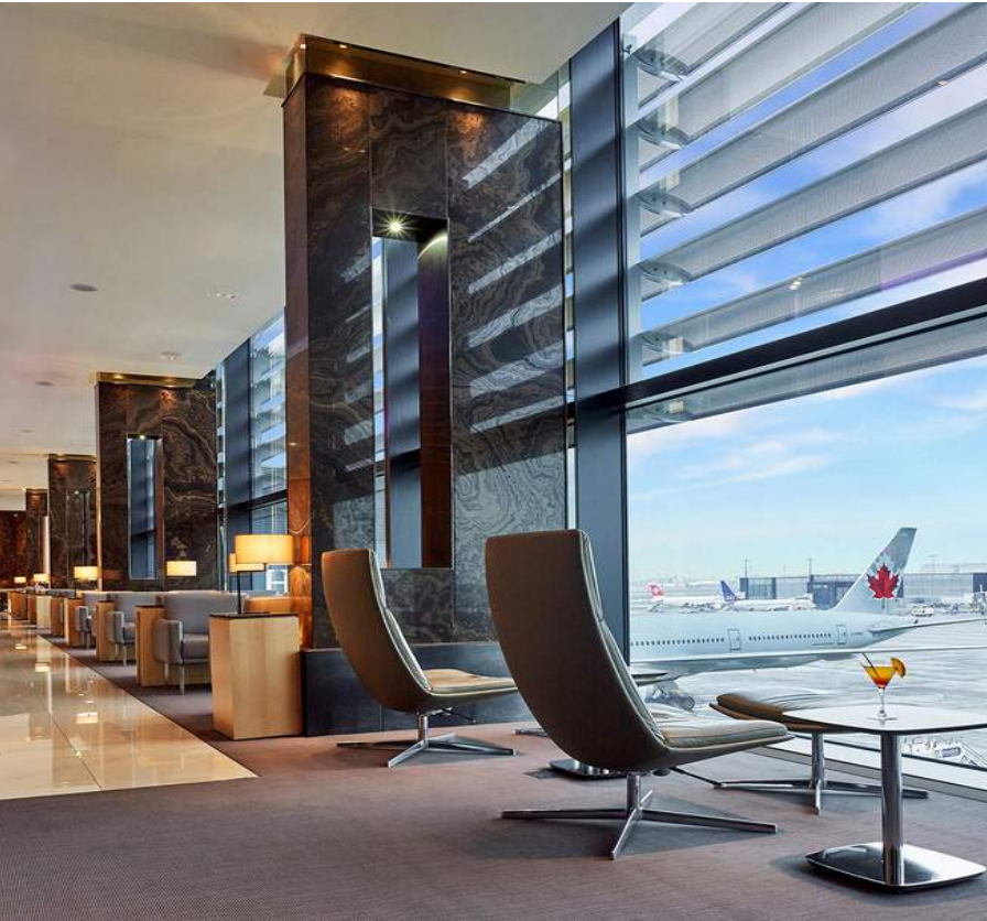
Eramosa marble pilasters featuring light weight cladding
