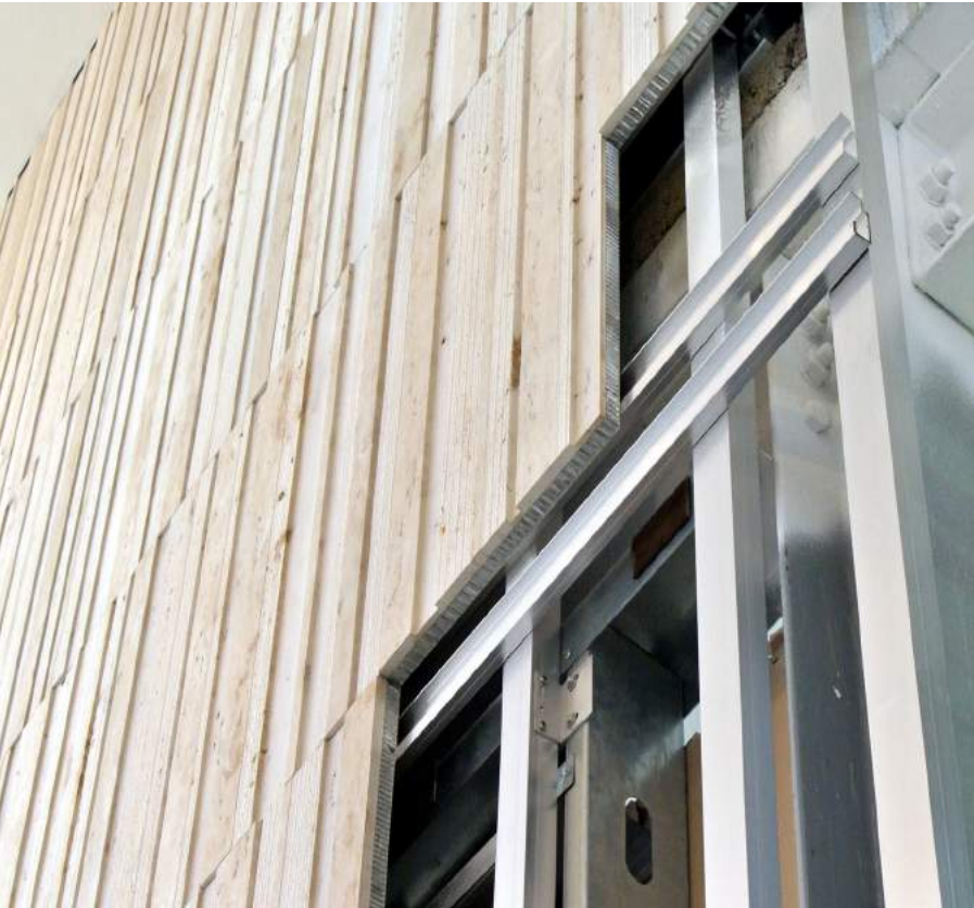
Jura Limestone fixed via aluminium sub-frame to steelwork
