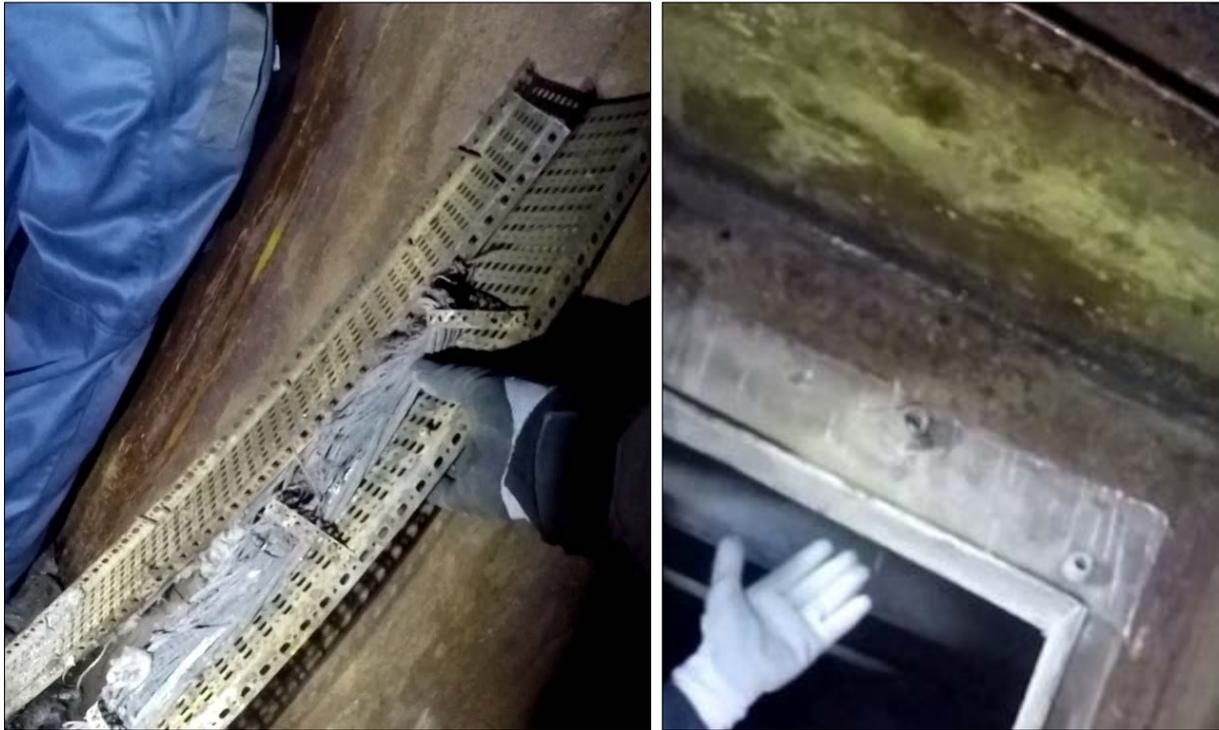
*Figure 11: Cable tray in storage room 1 and cable penetration between storage rooms 1 and 2*
