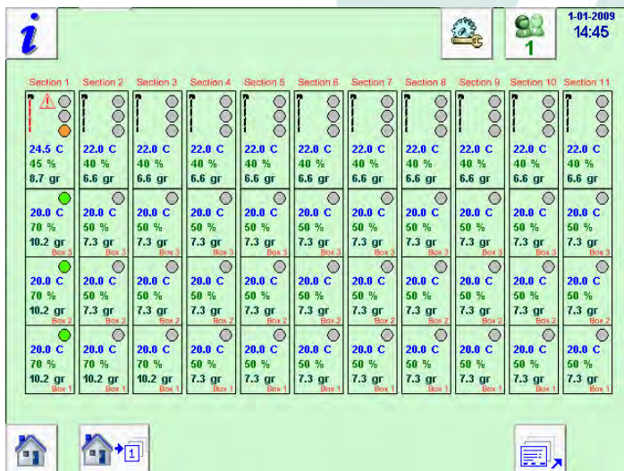
Example of an ABC HVAC-window showing controls
