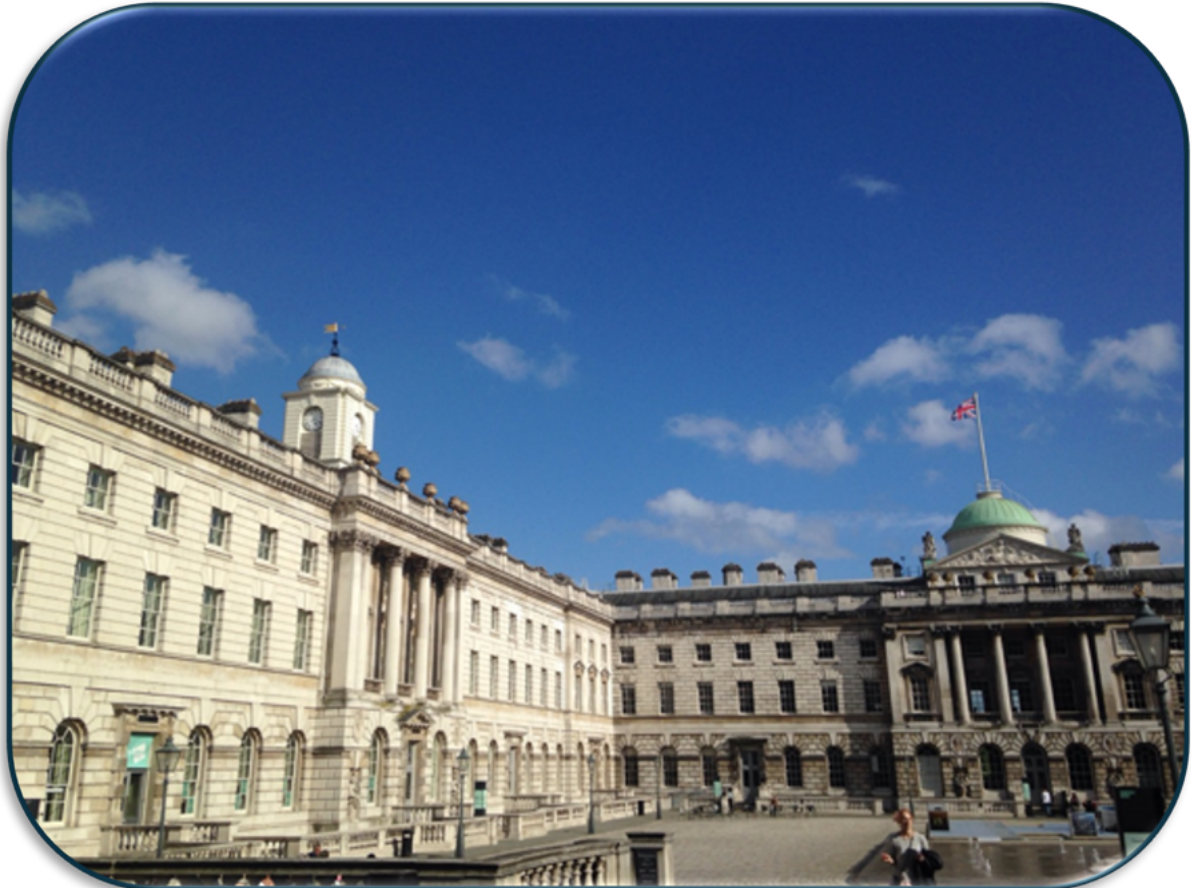
Strand campus, King's College London (Somerset House East Wing)
