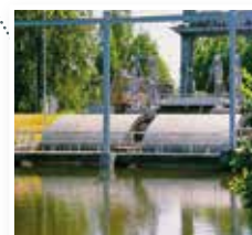
RAMNÄS, 1960 5,0 MW EFFEKT
