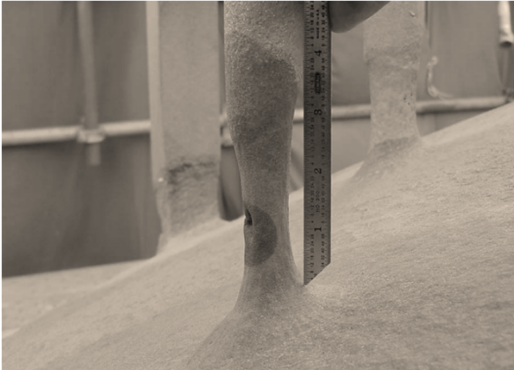
Figure 4-77 – CUI of nozzle on a top head.
