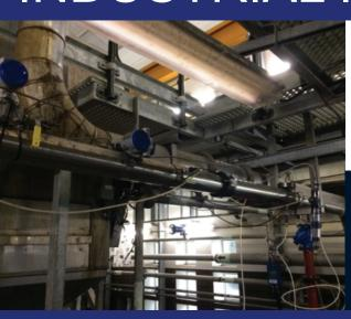
The Incipientus in-line rheology system was successfully installed in an integrated and operational WasteWater Treatment Plant (WWTP) environment.
