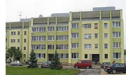
renovation of buildings
