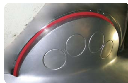
Step 6: Installed seals for runner blades
