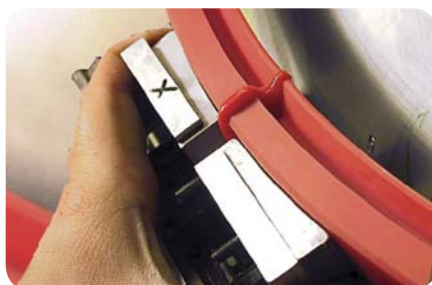
Step 3: Welding of aligned cross sections
