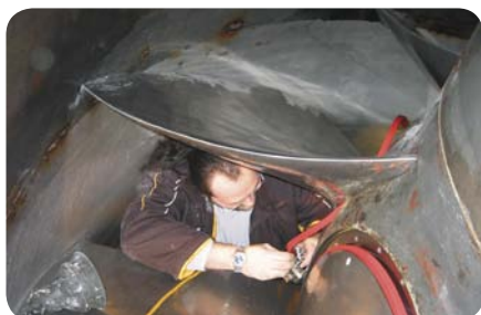
Step 1: Mounting of runner blade seals
