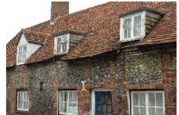
A traditional brick and flint cottage with small dormer windows and plain clay tiled roof. (Watlington)
