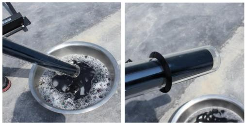
(5) Slowly insert the vacuum tube through the pipe holes on the water tank, then slowly put the bottom of the vacuum tube into the tube support, adjust the dustproof ring to a proper place.
