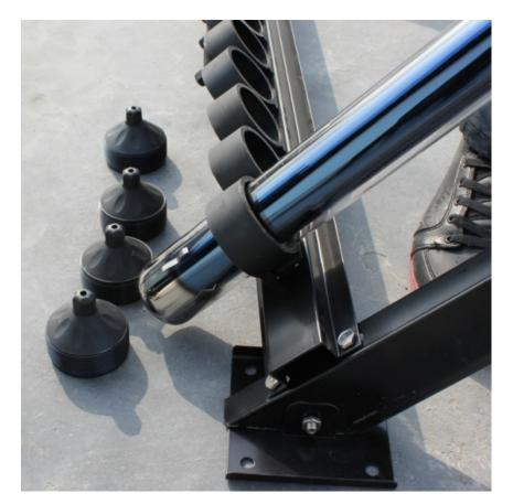
(7)Insert the condensing side through the blind pipe of the runner blind pipe, tighten the adjustable end of adjustable tube support.
