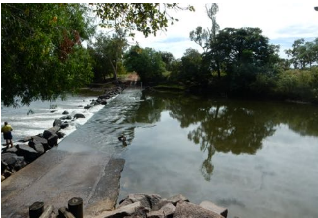
Cahill's Crossing. The Port to Arnhem Land.
