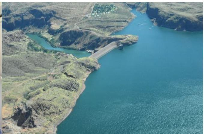
The Argyle lake dam wall
