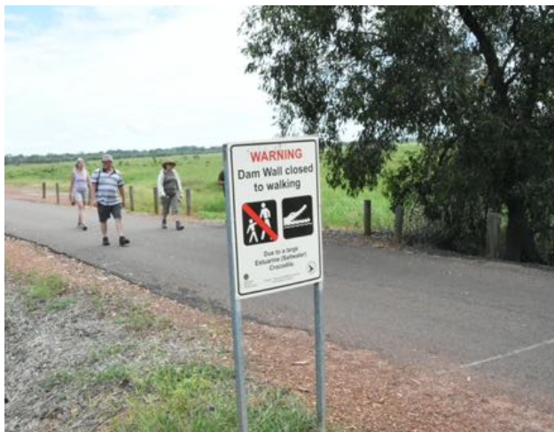
The fog dam dike
