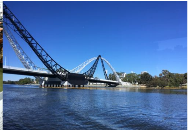
Ladies passed under the Matagarup Bridge
