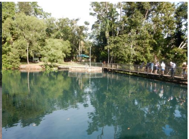
Howards Springs dam
