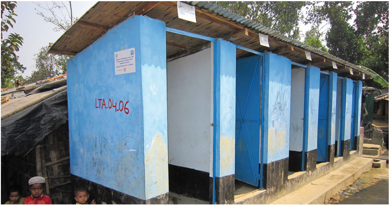
Figure 6: Toilets in Leda camp, provided by international aid project. The toilets are connected to a biogas plant.
