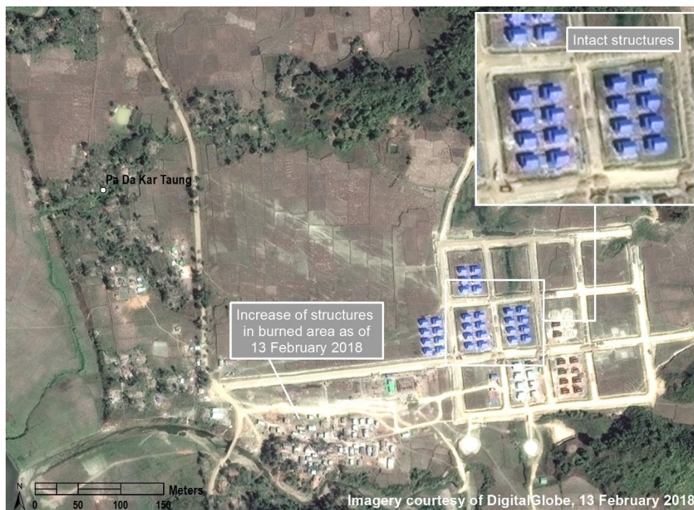
Image of Pa Da Kar Ywar Thit dated 13 February 2018 showing extensive new construction
