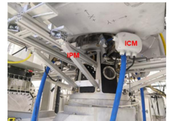
**Figure 3. Draft tube cone assembled with ICM & IPM systems.**
