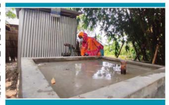
More than 300 double platform tube wells have been installed in different community places of flood prone areas of Gaibandha and Kurigram districts. During dry season, heads of these tube wells are set on the lower face and during flood, these are set on the upper face. As a result, affected people from the surrounding areas can collect safe water from these tube wells during flood and normal time as well.
