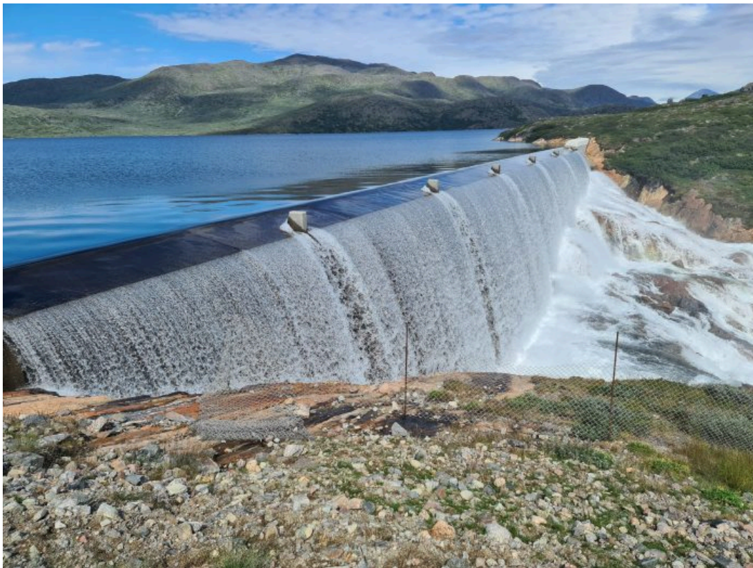
Dam of a small-scale hydropower station of 7MW in the South of Greenland, credit: Claus Andersen-Aagaard.
