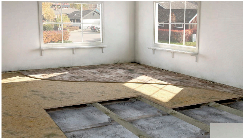
2. The concrete slab is cleaned of all organic material.
