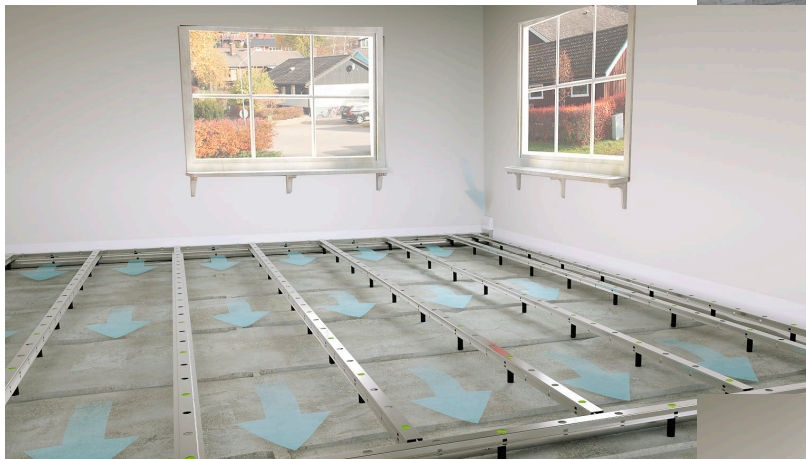
3. The Granab subfloor system with underfloor ventilation and insulation is installed.
