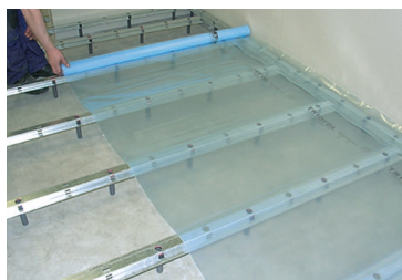
Installation, floating 22 mm chipboard
