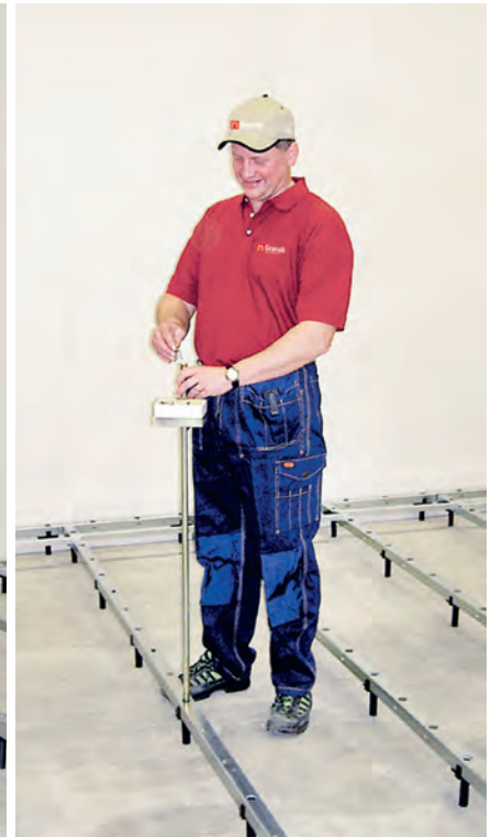
Installation pipe for concrete anchor.
