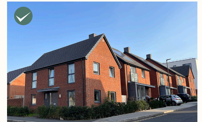
Active edges to all blocks - Dwellings that turn a corner should provide windows and/or doors to both frontages to avoid blank gables.
