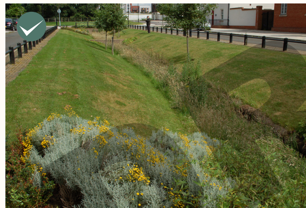
Linear Swale - Key feature of the character area, provides a SUDs solution to drainage and wetland habitat running through the heart of the development.
