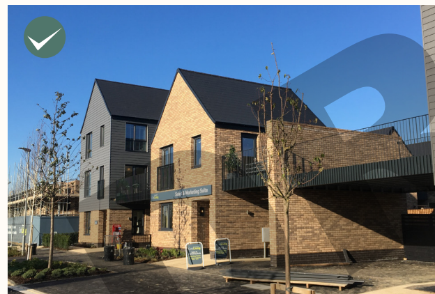
Raised deck amenity spaces provide open space for dwellings and reduce impact of driveway.
