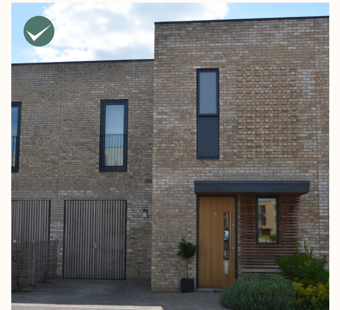
Roof forms - can include pitched or flat forms but should be consistent per street.
