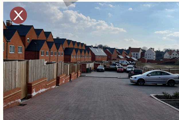
Parking - Should be integrated with the overall landscape of the street and overlooked by dwellings.
