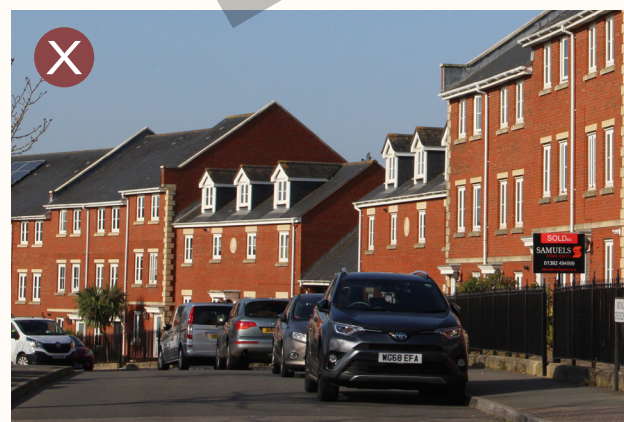
Inconsistent building typologies
