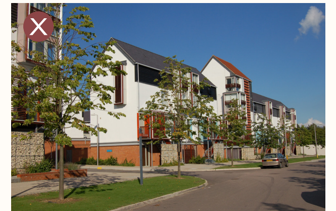
Inconsistent building form with mixture of stories.
