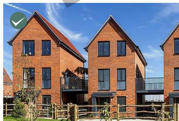
Raised deck amenity spaces provide open space for dwellings and reduce impact of driveway.
