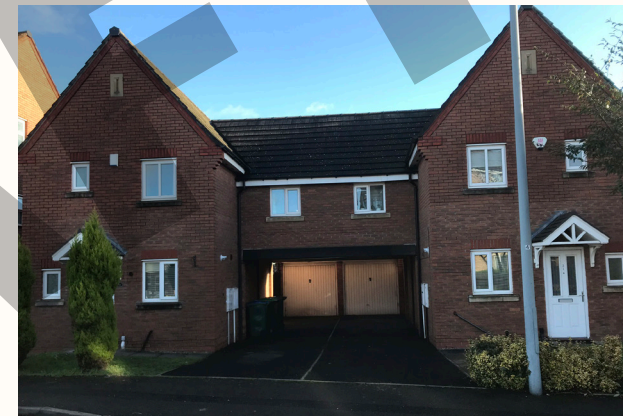
An example of semi-detached building with garage, Manifold Way. Materials include red brick. Brick lintels and grey tiled roofs.
