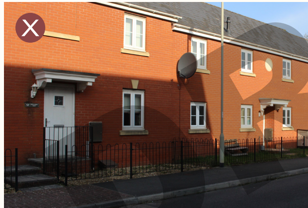
Hard landscaping to front of properties with fencing not acceptable.
