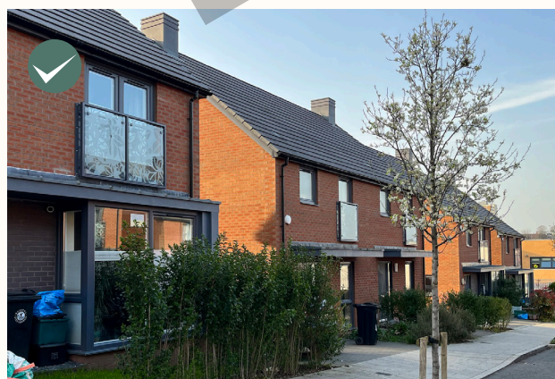
Consistency in building material in form to street.
