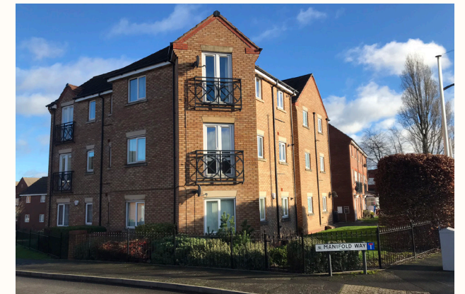
An example 3 story apartment building, Manifold Way. Materials include buff brick, stone colour lintels and ironwork on Juliette balconies. Boundaries include black railings.
