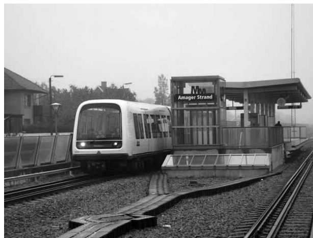
Amager Strand Metrostation
