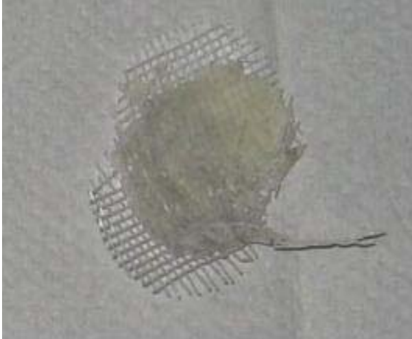
Picture 1: too narrow gap.
