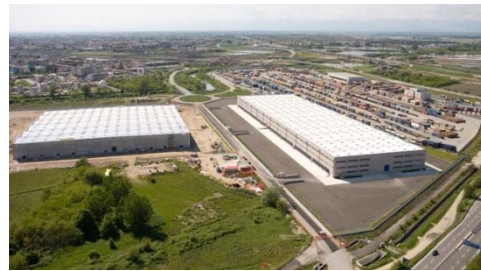
CIM Interporto Novara (Italy). Joint venture with local and provincial authorities.
