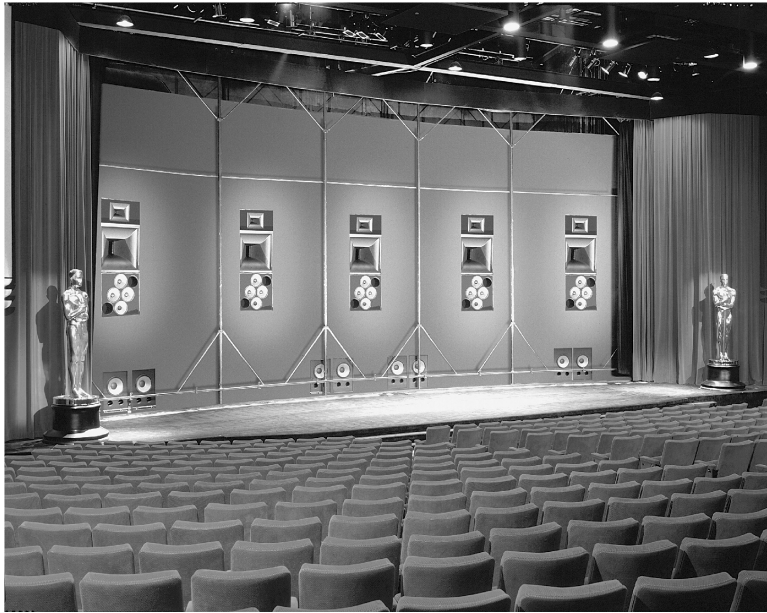
Figure 5. The Samuel Goldwyn Theater in the Academy of Motion Picture Arts and Sciences, Hollywood, California with the screen down and showing the five front channels and subwoofers, all JBL loudspeakers. Photo courtesy of JBL Professional; “Academy Award” and “Oscar” image © AMPAS ®. THX® Lucasfilm, LTD.
