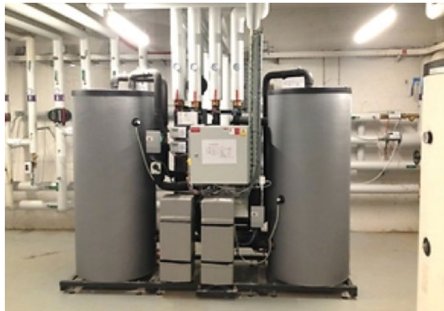
Figure 50 - Danfoss heat recovery unit (HRU) for heat recovery from a cooling system (Source: https://www.energy-supply.dk/announcement/view/103768/overskudsvarme_fra_koleanlaeg_bruges_som_fjernvarme )
