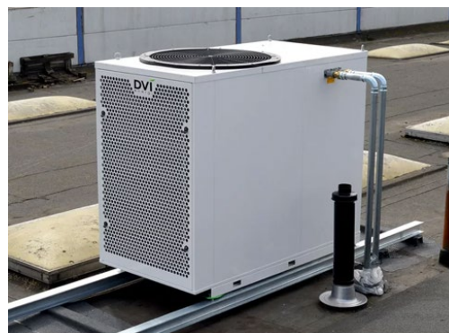
Figure 31 - the outdoor part of an air-to-water heat pump. The unit can be build as cascades to ensure larger effect. Source: https://dansk-energi-center.dk/varmepumper/store-varmepumper
