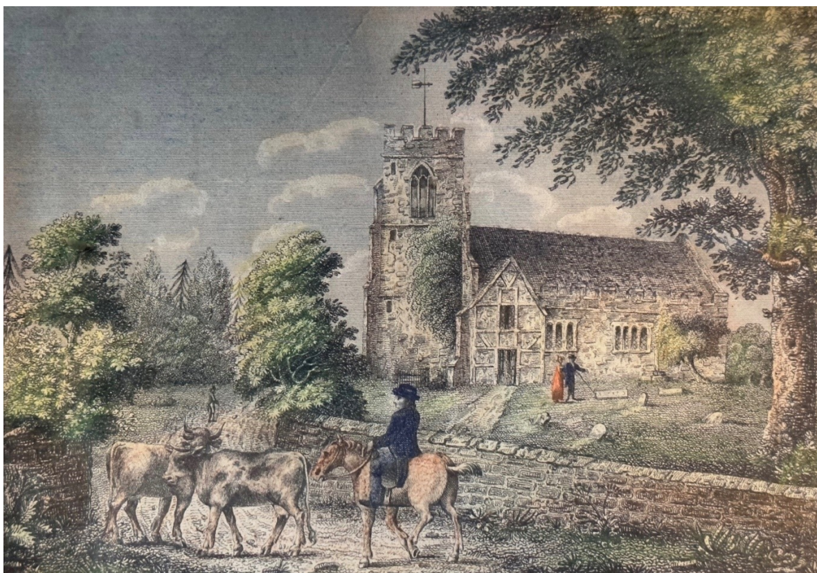
Figure 1 The Church at Eccleston during Aubrey's time as Rector.
