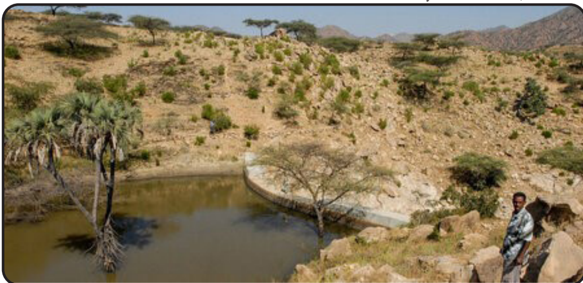
Of central importance in a region with unreliable rainfall the Jegar small dam
