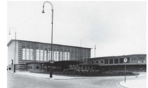
Station Amstel, ca. 1940
