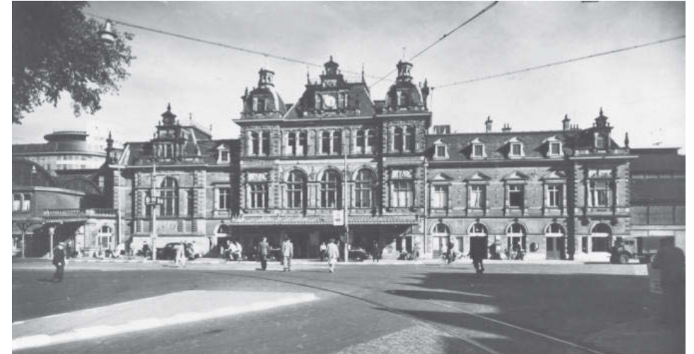
Station Den Haag Holland Spoor, 1891 (bron: htmfoto.net)
