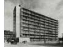
Bergpolderflat architect: W. van Tijen
