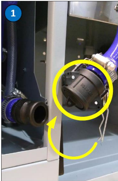
Disconnect the water inlet.
