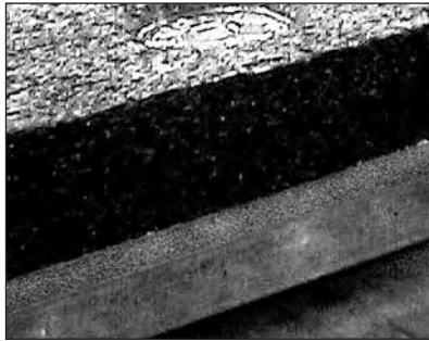
Fiber-Free liner on single duct terminal unit.
