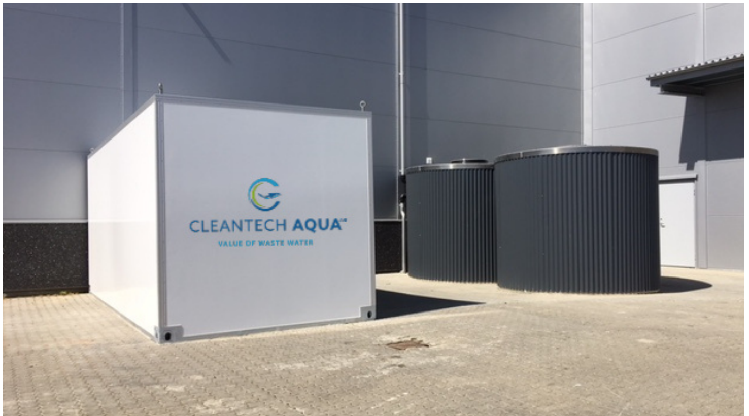
An over-ground wastewater recycling system (on the left), a rainwater harvesting tank (in the middle) and a sludge/settling tank (on the right).
