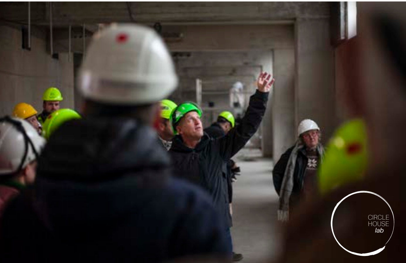
Image: Studytour at demolitionsite © GXN Innovation
