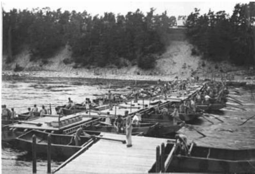
125 m long pontoon bridge over Dalälven, at Laxön; load capacity 15 tons. The picture was found on the Internet.
