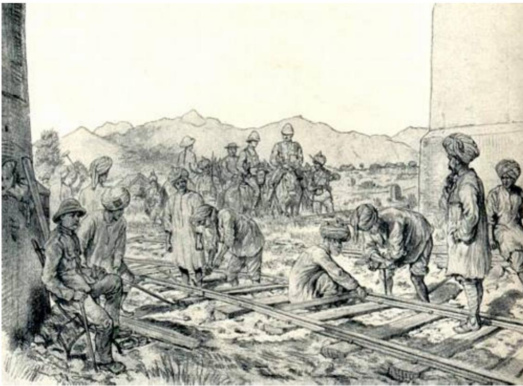
Indian soldiers and civilian workers repair a railway line in China, approx. 1900 6 . _
