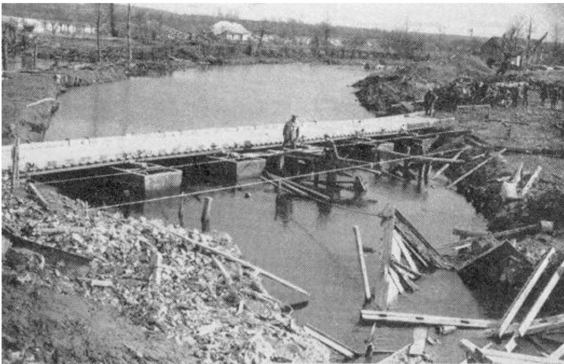
Same bridge, seen from the opposite bank.
