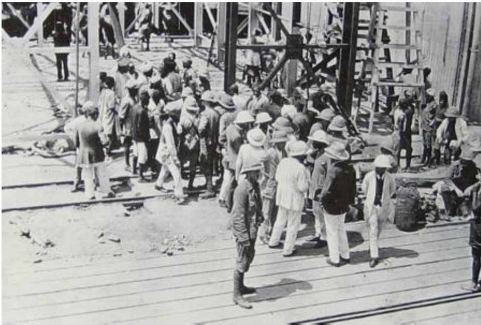
The shipping dock in Kisumu, 1915.
