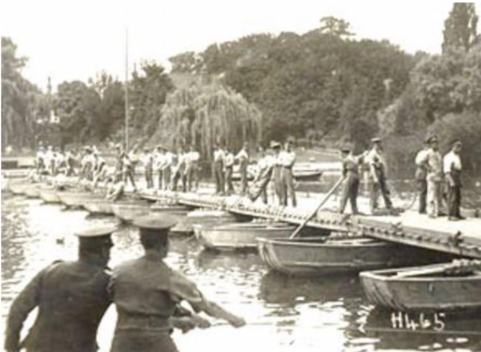
The Kent (Fortress) Royal Engineers carrying out bridge-building exercises.
