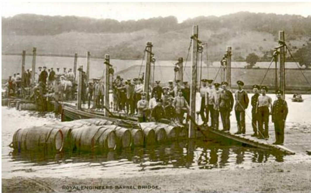
Royal Engineers Barrel Bridge, 1916.
