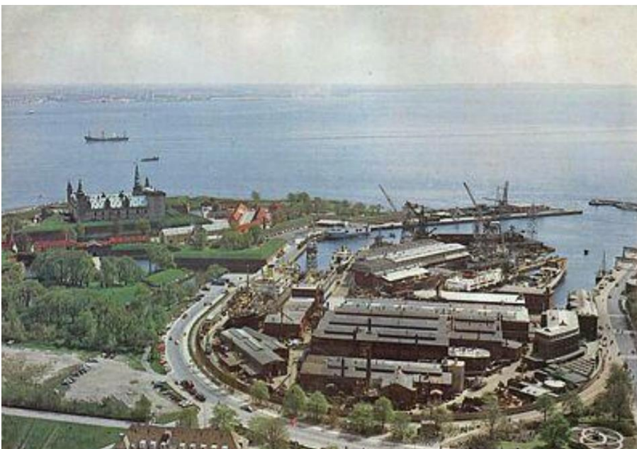
Helsingør Harbour, seen from the air (1965). From the Handels og Søfartsmuseet's digital photo archive .
