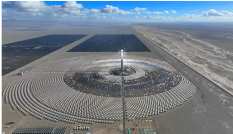
Gansu Jiuquan 750 MW CSP-PV coupled power generation project
