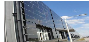
Solar PV integrated building
