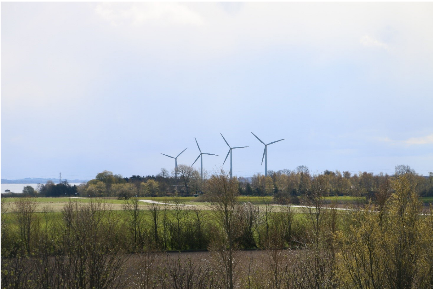
Figure 9: Distributed wind in forest area in Torup, Denmark (cc). Øyvind Holmstad
